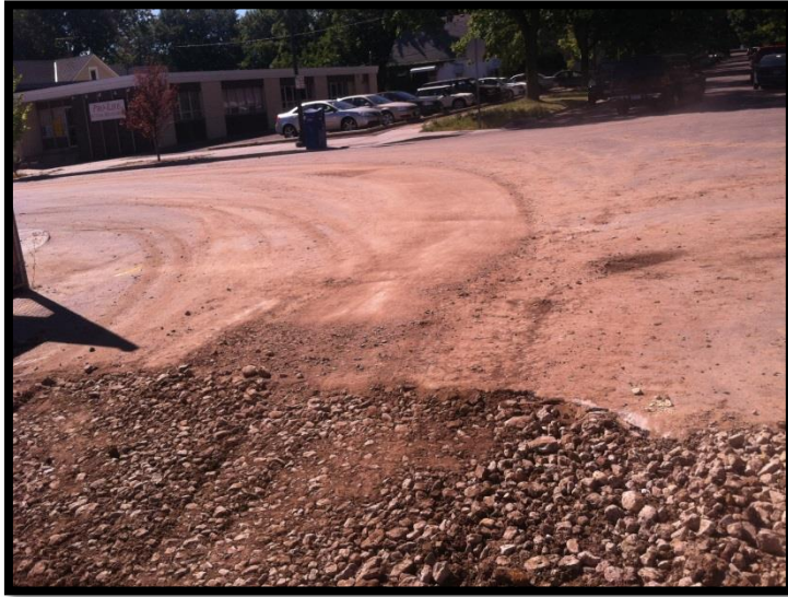
Sediment tracking on pavement.
